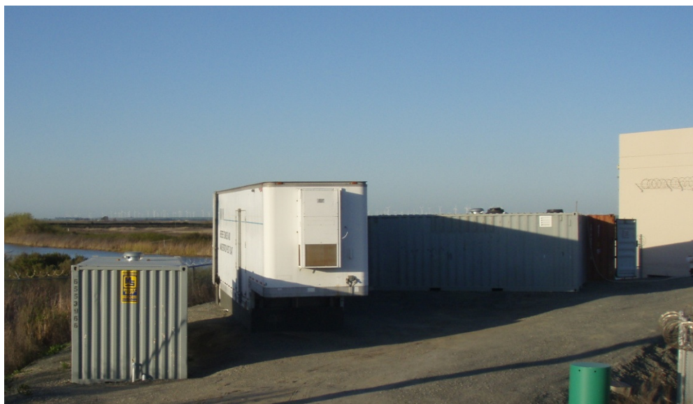
Figure 2-3: Pilot Plant Site
