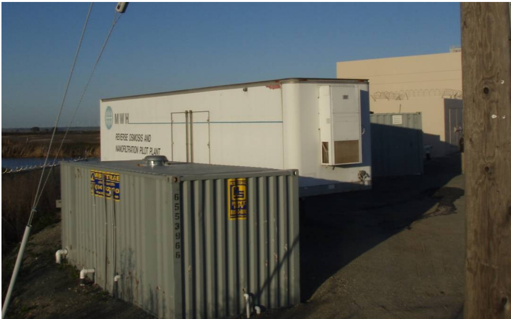
Figure 3-3: View of Pilot Plant Site at Mallard Slough Pump Station.
