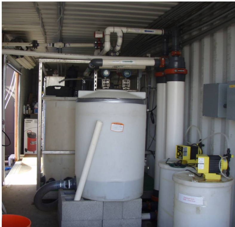
Figure 3-6: Pressurized UF System
