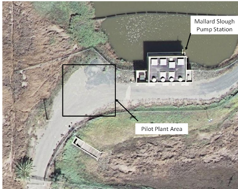
Figure 3-1: Pilot Plant Area
