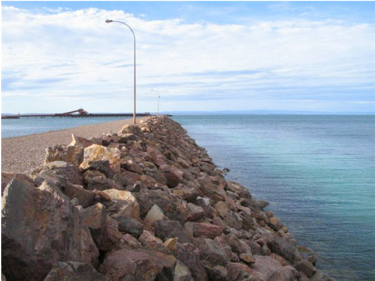
Figure 3-12. Porous Dike (Jetty)
