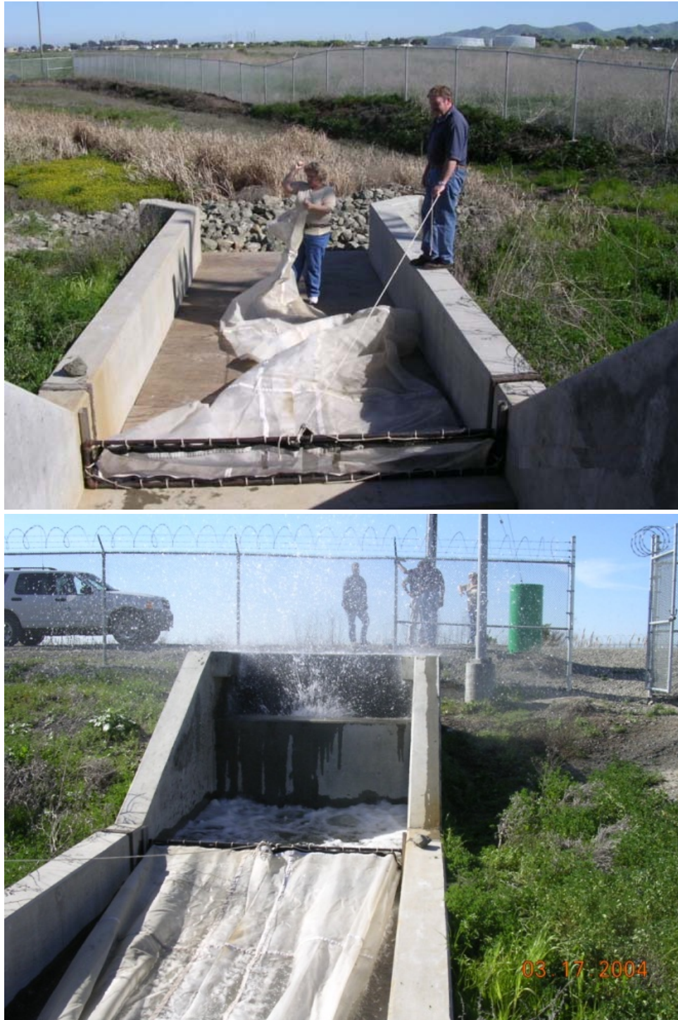
Figure 3-3. Entrainment sampling gear used during the Bay Area Regional Desalination Project pilot plant entrainment study for surveys conducted in February and March 2009.
