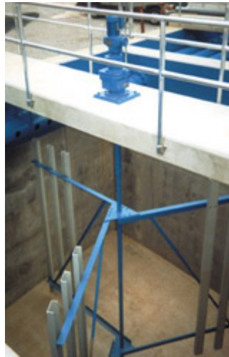
Figure 4-7 Typical Vertical Paddle Flocculator
