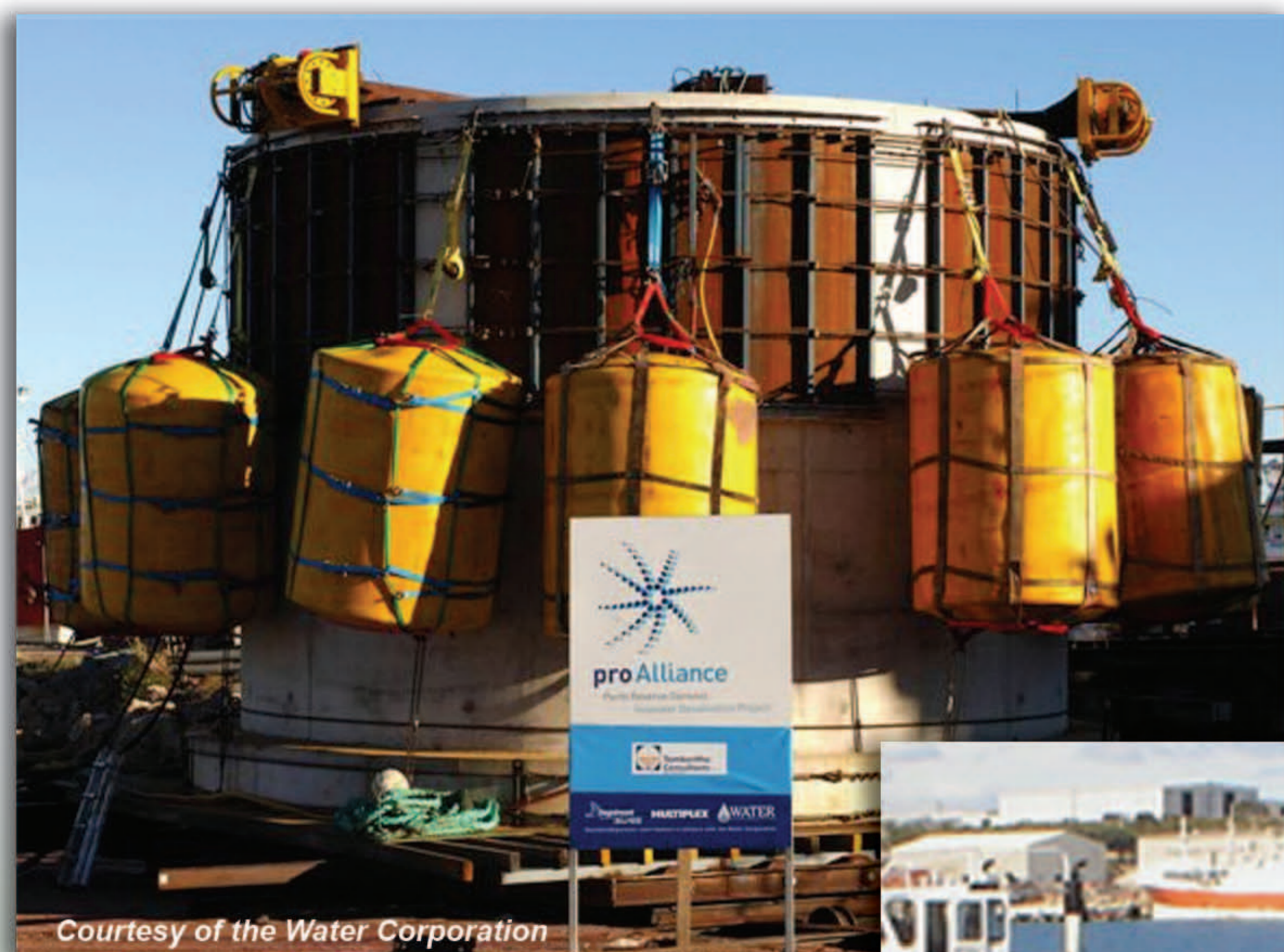
Seawater intake being installed
